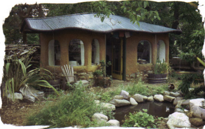
This garden studio in Northern California, built by Cob Cottage Company and the Permaculture Institute of Northern California, demonstrates cob's potential for rounded, sculptural shapes. (Photo by Michael Smith)
