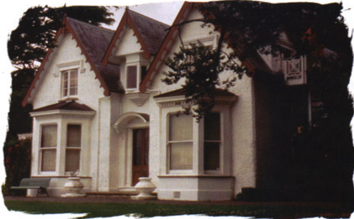
"Broadgreen," a Victorian cob mansion built in Nelson, New Zealand, has survived two major earthquakes with no apparent damage. Quakes that occurred in the 1870's and in 1931 destroyed neighboring brick buildings. (Photo by Ianto Evans)
