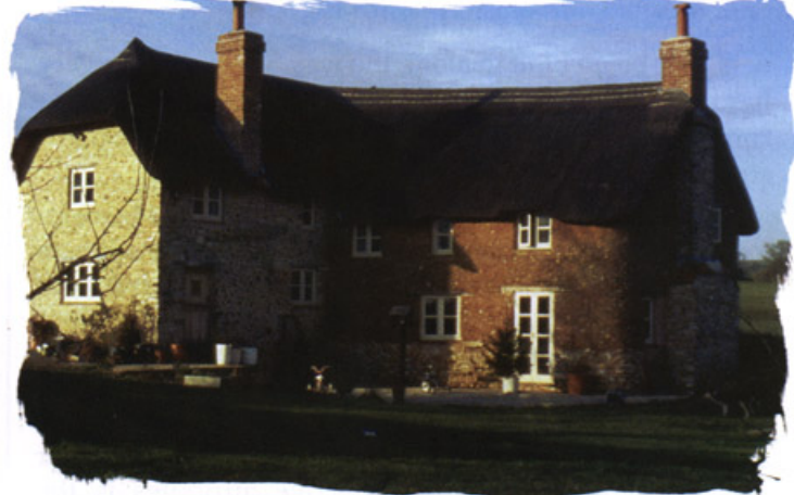
This four-bedroom cob and stone farmhouse, built by Kevin McCabe in 1994, marked the beginning of the cob revival in England. (Photo by Ianto Evans)
