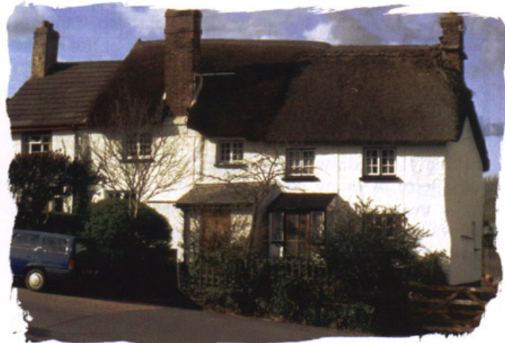
These 16th-century row houses with thatched roofs are typical of the approximately 2,000 cob houses that remain in use in the County of Devon, England. (Photo by Ianto Evans)
